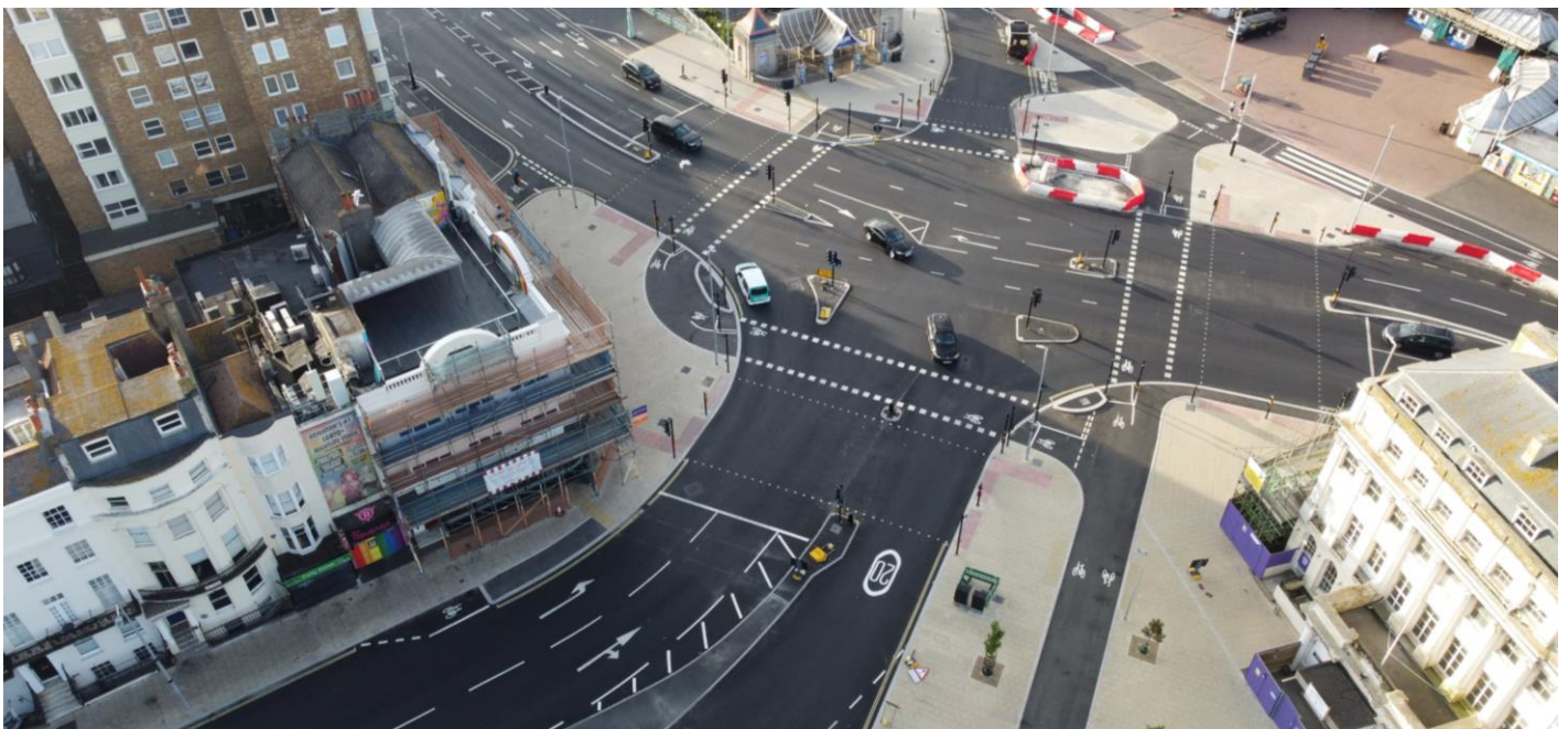
New aquarium junction is now operational – work is continuing to link traffic lights to nearby junctions
